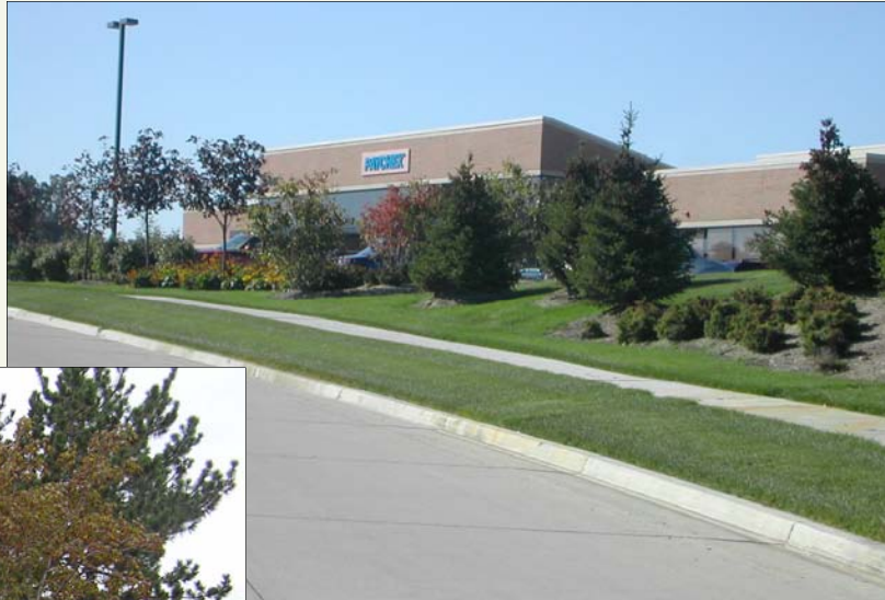
Landscaping can be used to feature a building (left), as well as screen it (above).
