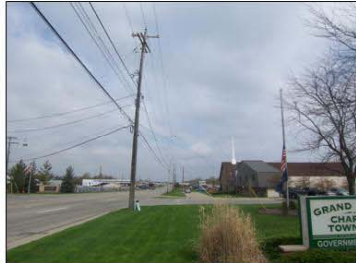
A. Overhead utilities within Right-of-Way
