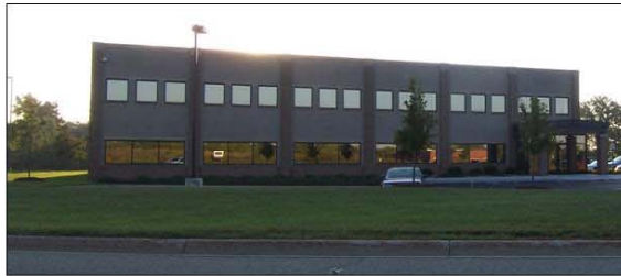
A. 2-story R&D building, limited front yard parking
