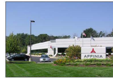
C. 1-story R&D building, limited front yard parking
